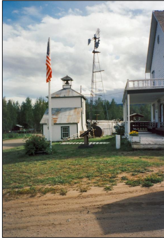
(Community Water Pump House – Eagle, AK)
