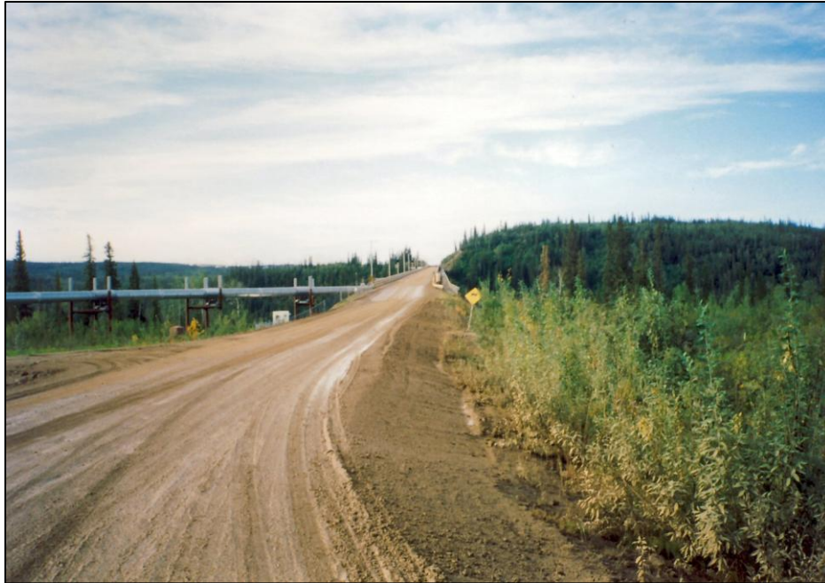
(Yukon River Bridge – note the grade)
