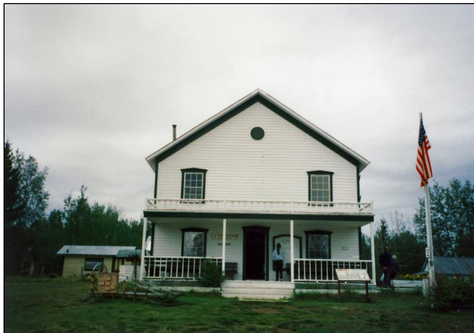
(Wickersham Court House –Eagle, AK)
